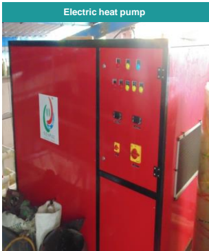
Electric heat pump
